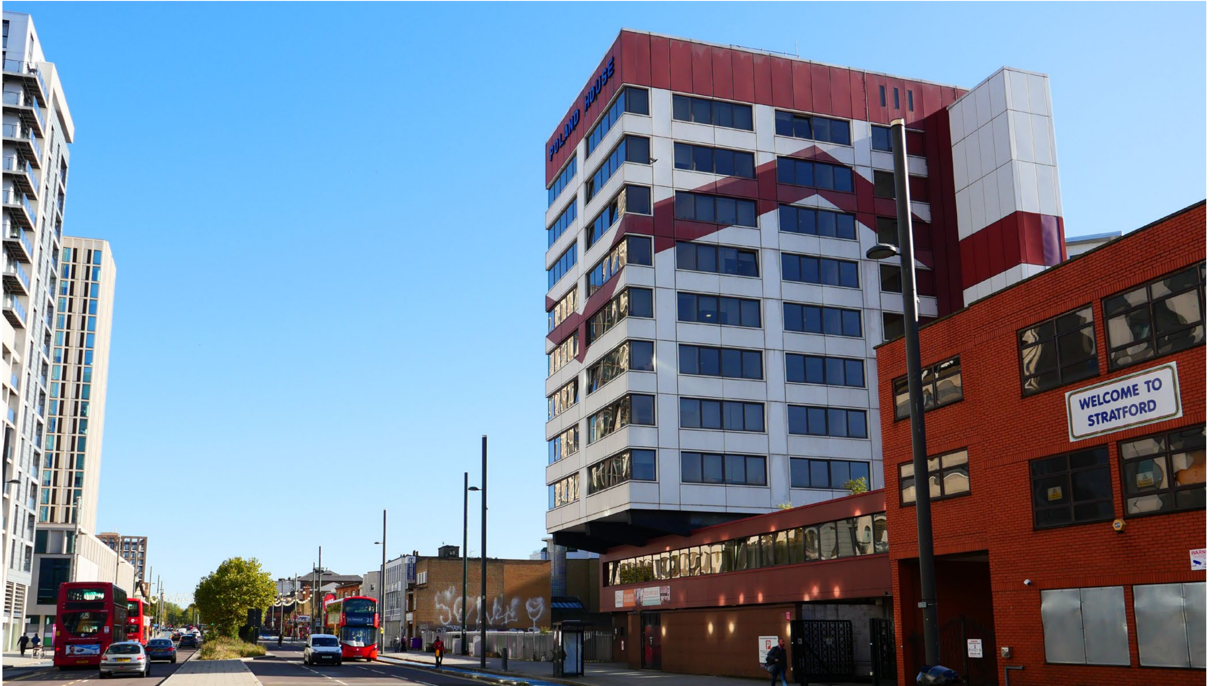
Photo of the site.
